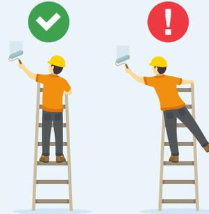
Ladder should be positioned closely to avoid overreach.
