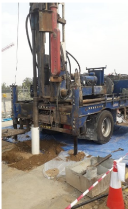
Groundwater well being installed (left) and sampled (right)
