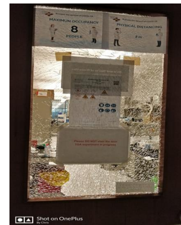
Damage to window in the service corridor door.
