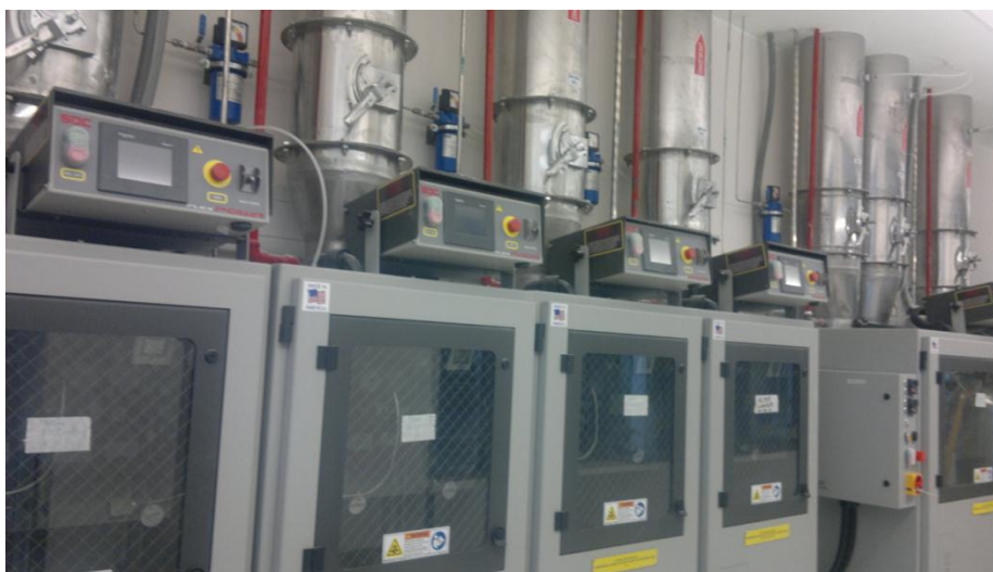
Fig.1 Gas cabinets provided for non-toxic gases
