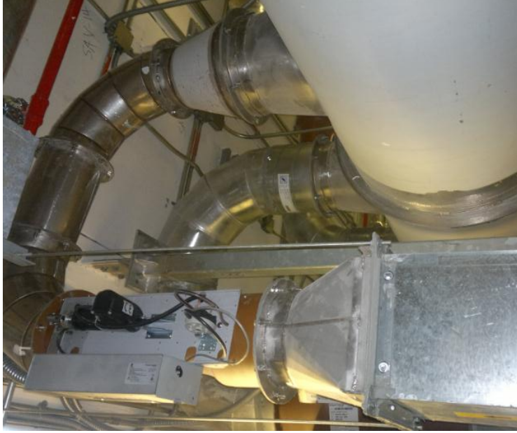
Fig.1 Phoenix valve and attenuator provided for single cabinet
