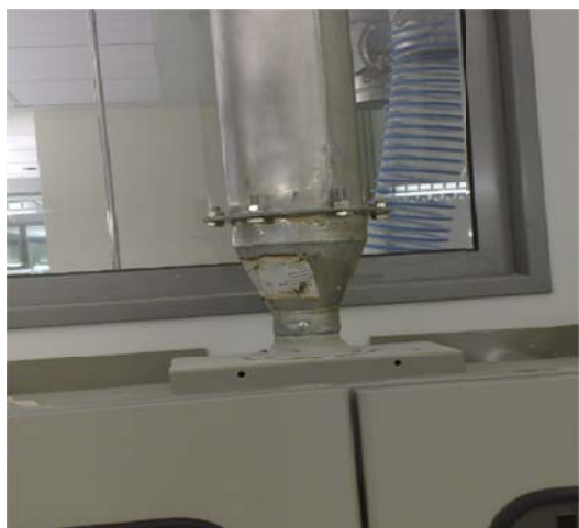
Figure 13: Exhaust connection for vented chemical storage cabinets
